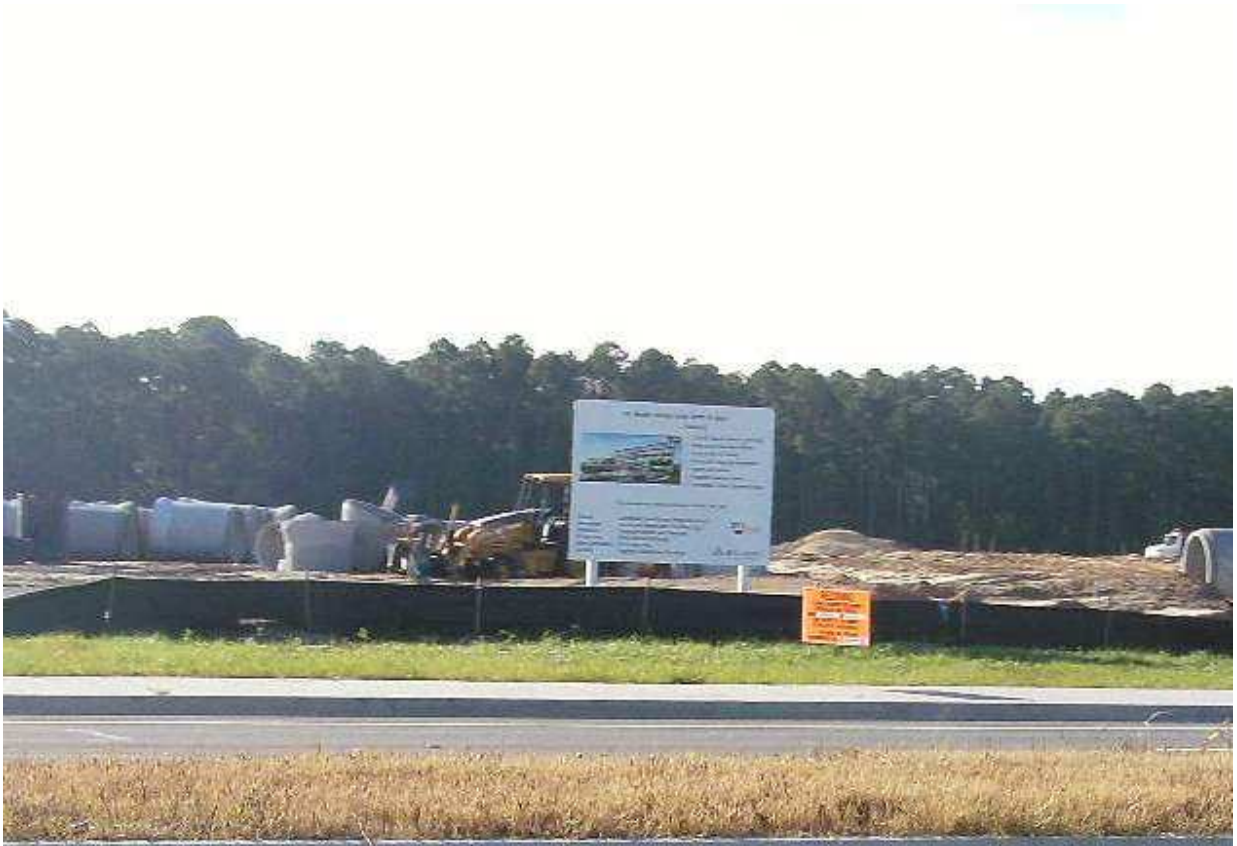
Site is under construction
